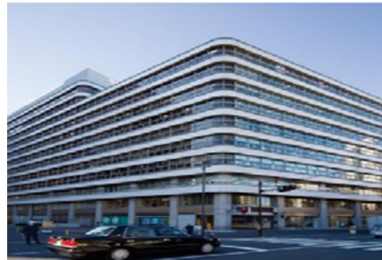
Figure 7-1. Appearance of Nippon Building
